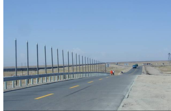
Heat pipe subgrade
