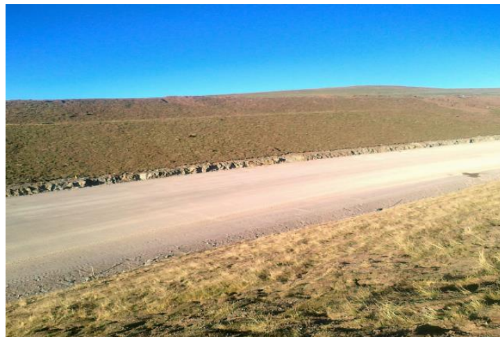
Sod protection cut slope
